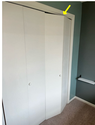
Upstairs bedroom closet door does not fully close.
