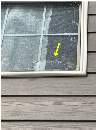
Large hole in window screen on East side of home.
