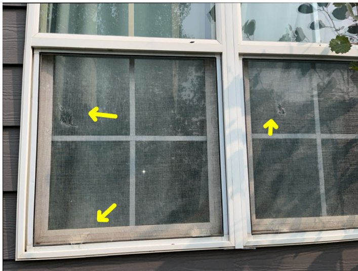
Large holes in window screens on South side of home.
