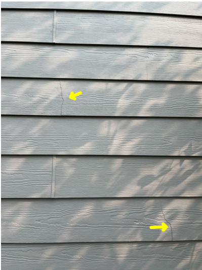
Cracked siding planks on South side of home.
