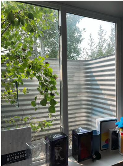
Basement window screens missing.
