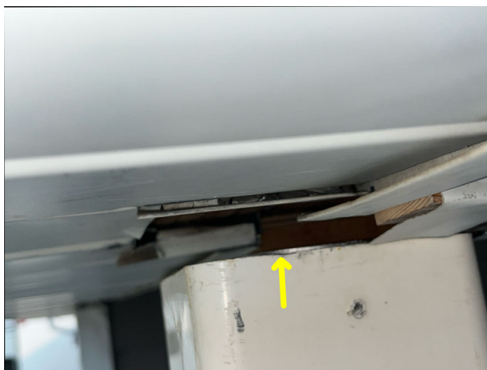
Support post at front entrance appears to have settled. Not supporting roof above.
