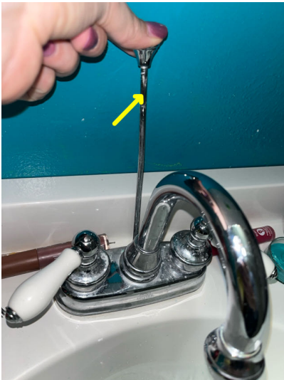
Sink drain plug needs repair or replacement.
