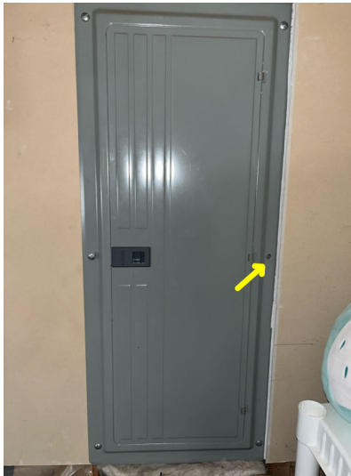
Panel cover screw missing.
