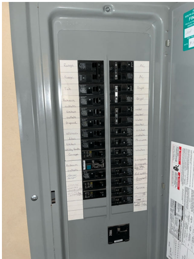
Breakers marked at main panel.
