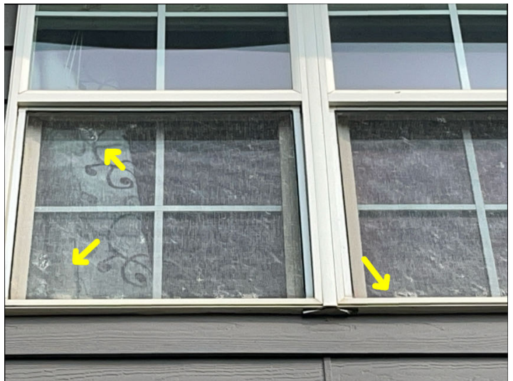
Holes in window screen on upper level window on South side of home.
