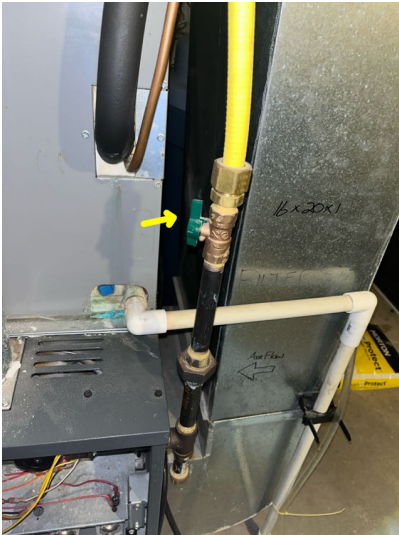
Gas line with shut off valve located at front of unit.
