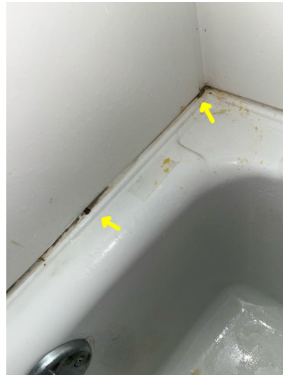
Organic substance growing on tub caulk. Recommend removing and re-caulking.
