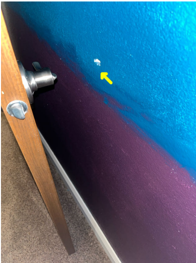
Basement bedroom door stop missing. Previous wall damage noted.
