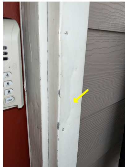
Damage to trim around front entrance.
