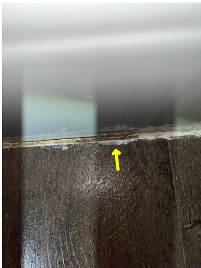
Tub - floor junction needs caulk.
