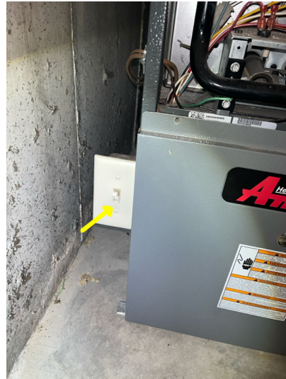
Power source located on bottom left of unit.
