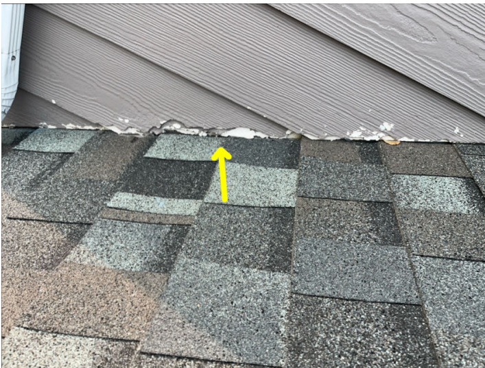
Siding damage on East side of home above garage roof.
