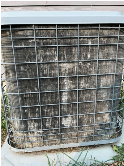
Dirt and damage noted to AC unit coils.
