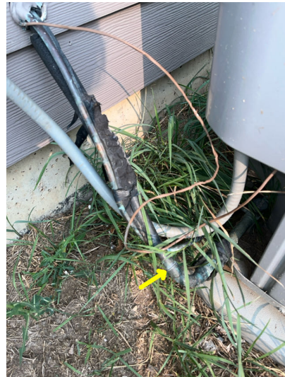
AC line set insulation damaged.
