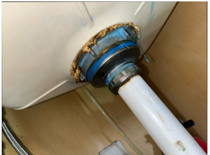
Previous repairs noted below kitchen sink. Dry at time of inspection. Monitor.
