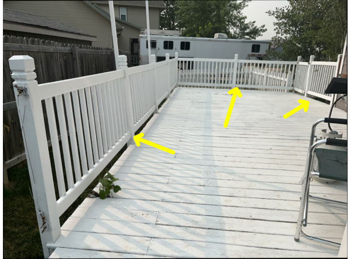
Railings loose around entire deck.
