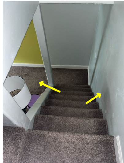
Hand rail and guard rails missing.
