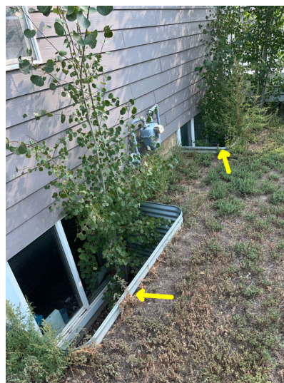
Open window wells below grade on South side of home.
