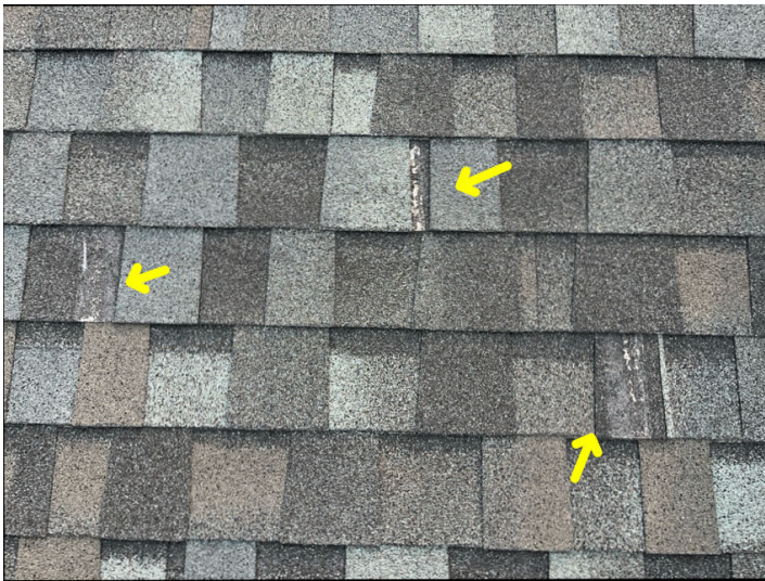
Shingle damage on West facing roof.
