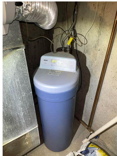
FYI: water softener system located next to furnace.
