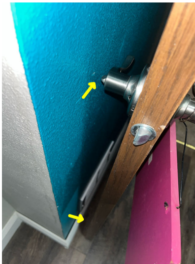
Basement bathroom doorstop missing. Previous wall damage noted.
