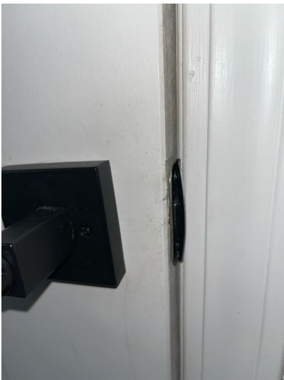
Half bathroom door does not shut and latch.
