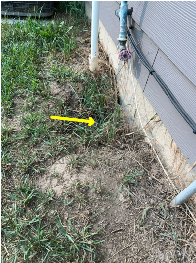
Low area of grading on East side of home.
