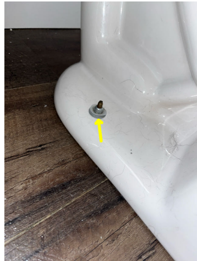
Toilet anchor bolts should be capped for safety.
