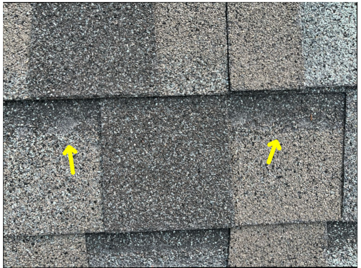
Shingle damage on West facing roof.
