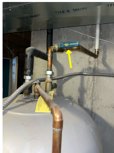
Water supply lines with shut off valve located on top of unit.
