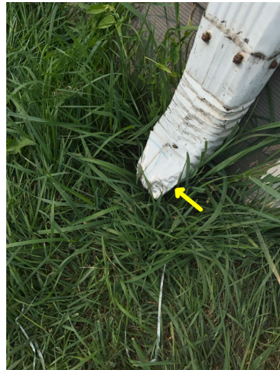
Downspout at Northeast corner of home drains near foundation.
