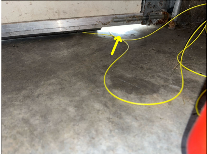
Air and light entering at corners of vehicle garage door.
