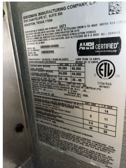
Model and serial number of furnace. Manufactured 2014. 64,000 BTU output.
