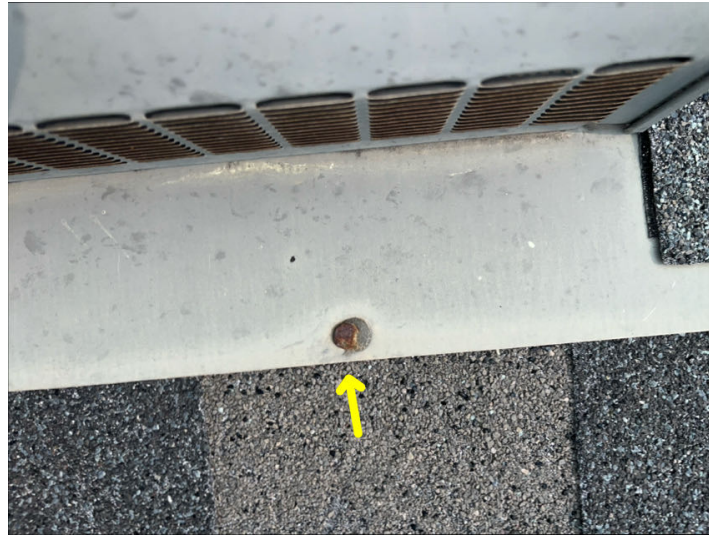
Exposed nails on roofing material.
