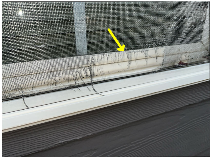
Large holes in window screen on West side of garage.
