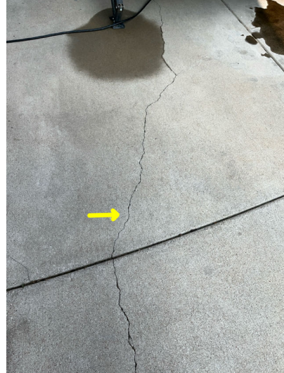
Minor cracks at top of driveway.
