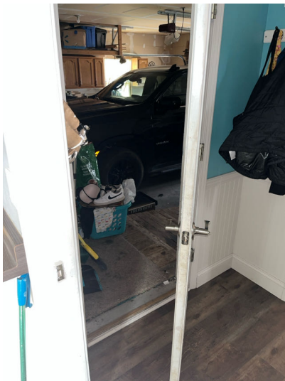
Garage-house door does not close automatically.
