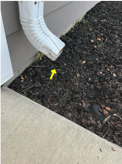
Downspout at front of home drains near foundation.
