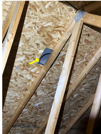
Roof ventilation appears adequate.
