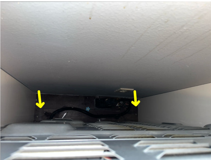
No anti-tip brackets installed behind range.
