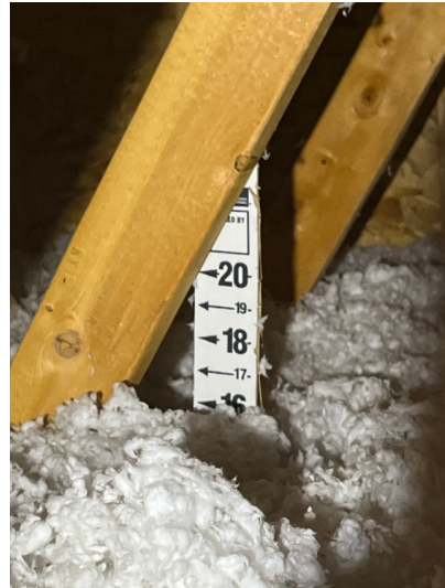
Blown-in fiberglass insulation averages about 14-16 inches in depth.
