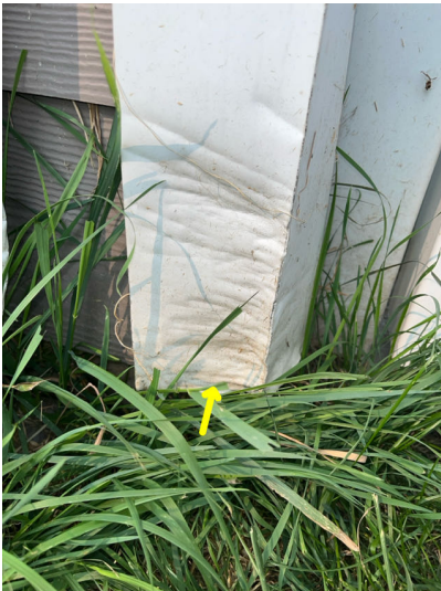
Northeast corner trim damaged.
