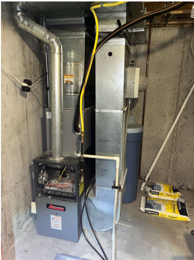
Gas furnace located in basement utility room.
