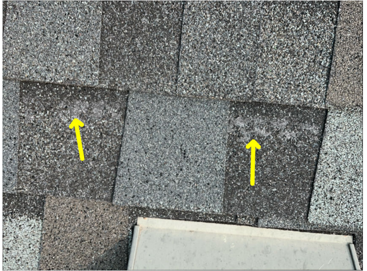
Shingle damage noted on South side of roof.
