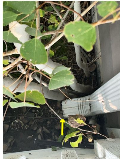
Downspout at Southeast corner of home drains near foundation.
