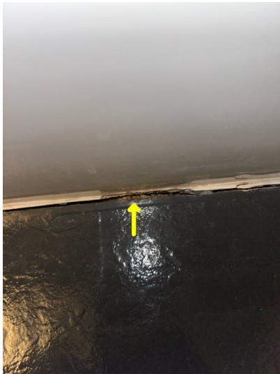
Tub - floor junction needs caulk.
