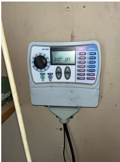
Sprinkler system controls located in garage.
