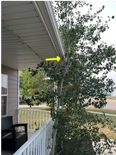
Tree at front of home rubs on shingles and gutter. Trees growing in window wells next to foundation.
