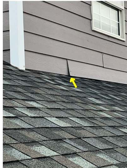
Siding board loose at front of home above roof line.
