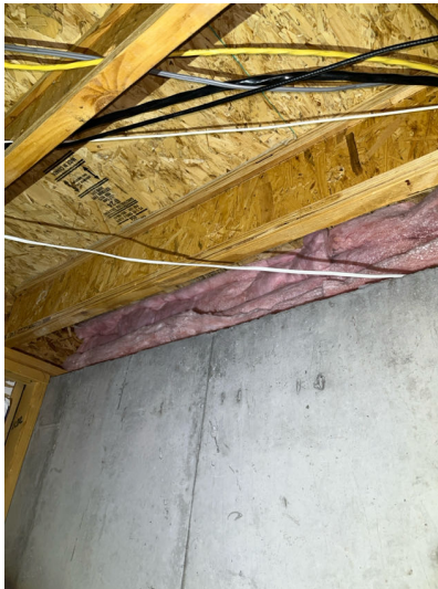
Manufactured I-joists and insulation at sill plate.
