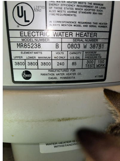
Model and serial number of water heater. Manufactured 2003.
