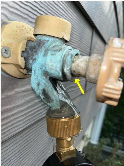
Water spigot on West side of home leaking at valve seal.
