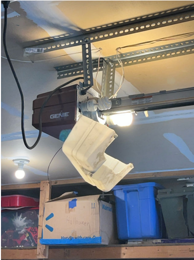
Cover loose on vehicle garage door motor.
