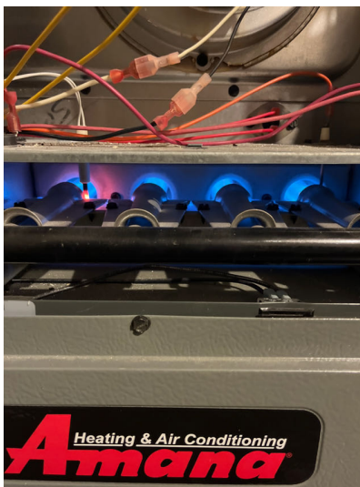
Burners firing.
