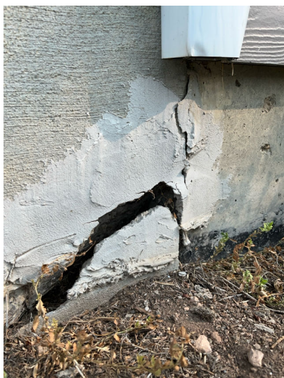
Large crack in South side of front patio.
