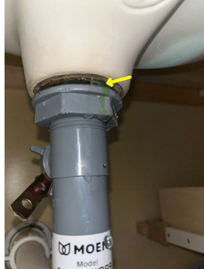
Leak in drain line below sink.
