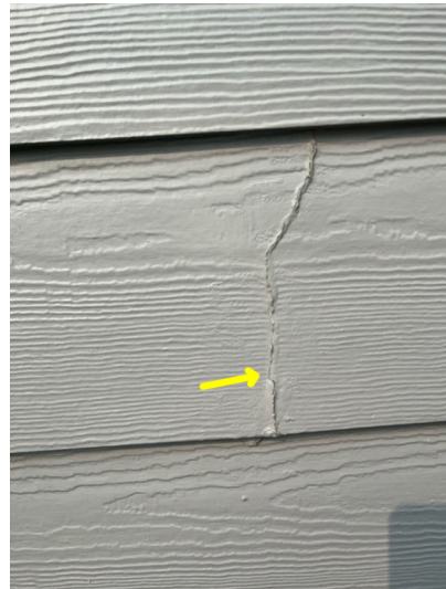
Crack in siding on East side of garage.
