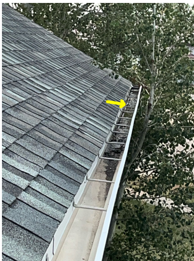
Gutters full of debris at front of home.
