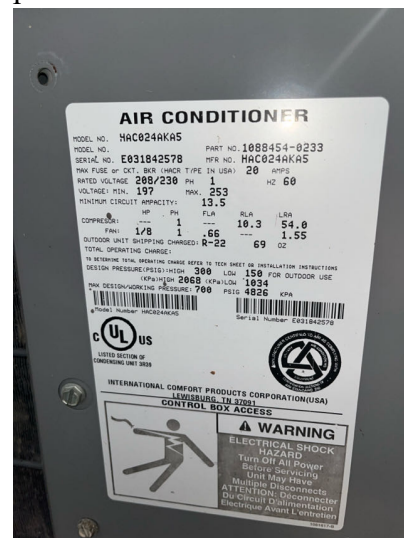
Model and serial number of AC unit.
