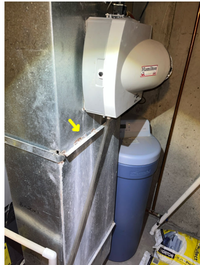
Evidence of previous leak behind humidifier.
