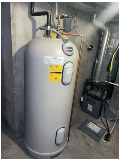
Electric water heater located in basement utility room.
