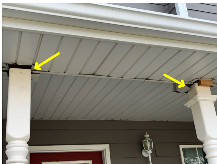
Front entrance support posts appear to have settled.
