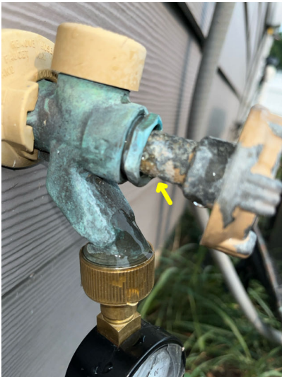
Water spigot on East side of home leaking at valve seal.
