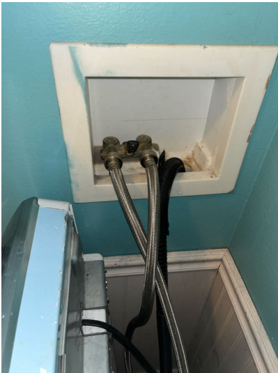
Washer supply lines and drain line located in wall to left of unit.
