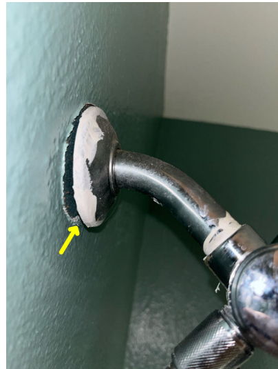
Shower head flange not secured to wall.
