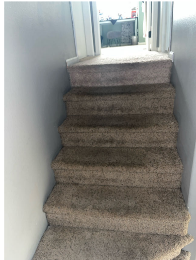
Stairway to upper level. Hand rail missing.
