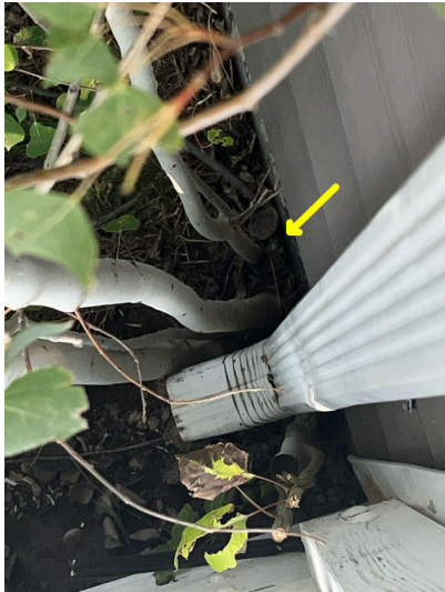
Tree growing next to foundation at Southeast corner of home.
