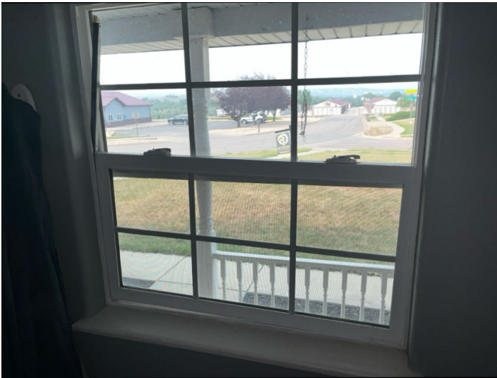
Window in front entryway does not stay open.
