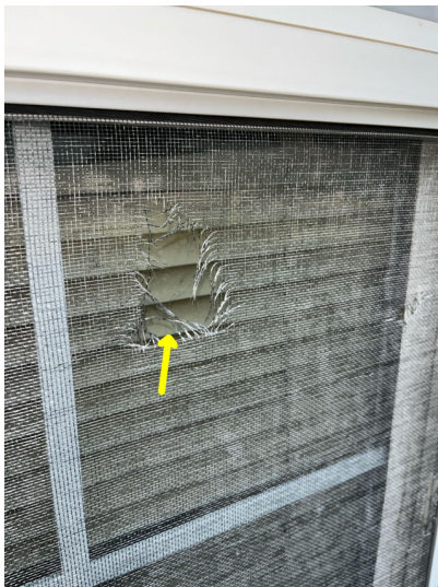
Large holes in window screens on West side of garage.
