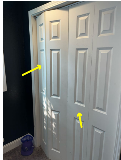
Basement bedroom closet door does not fully close. Door handles missing.
